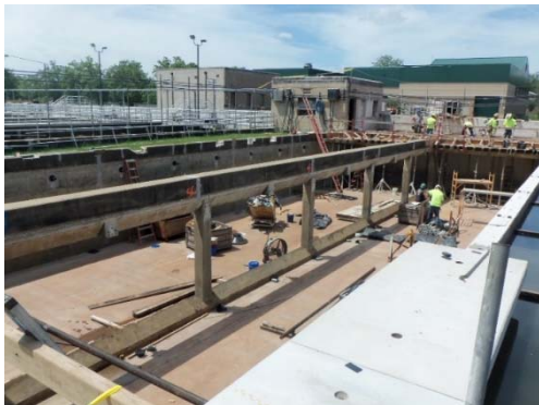
Primary Clarifier 4 —During Construction
