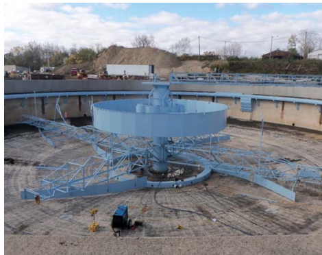
Clarifier 7 —New mechanism and bridge
